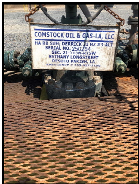
Derrick 21 HZ #3 Well Head
