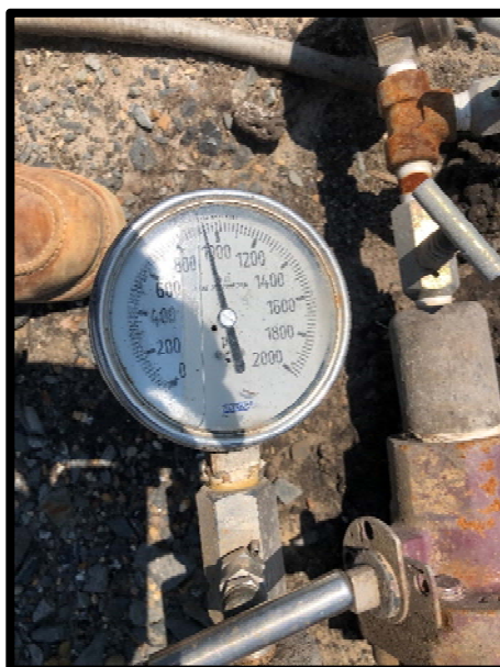
Gauge for well surface casing
