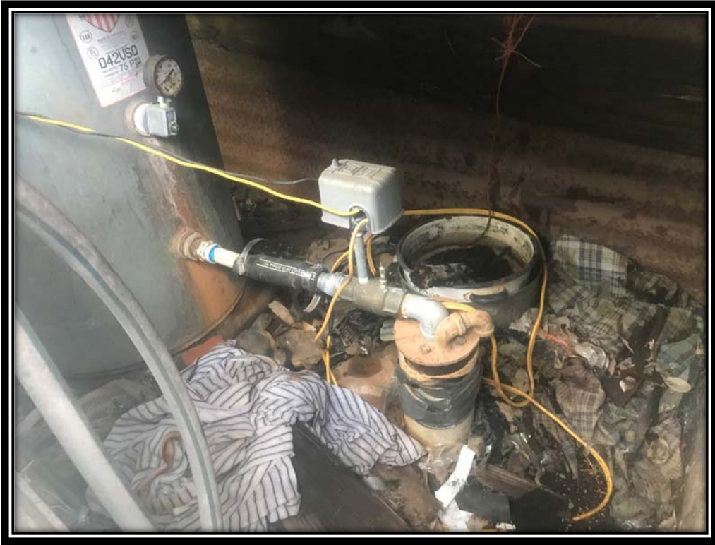
Cleon Bryant-9769Z water well with pump and tank
