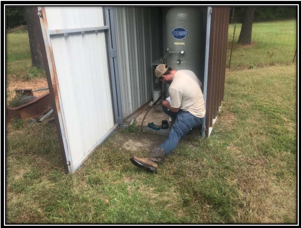
Pump Shed, Purging and collection point
