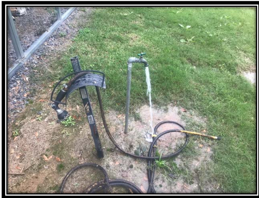
Purging and sampling point
