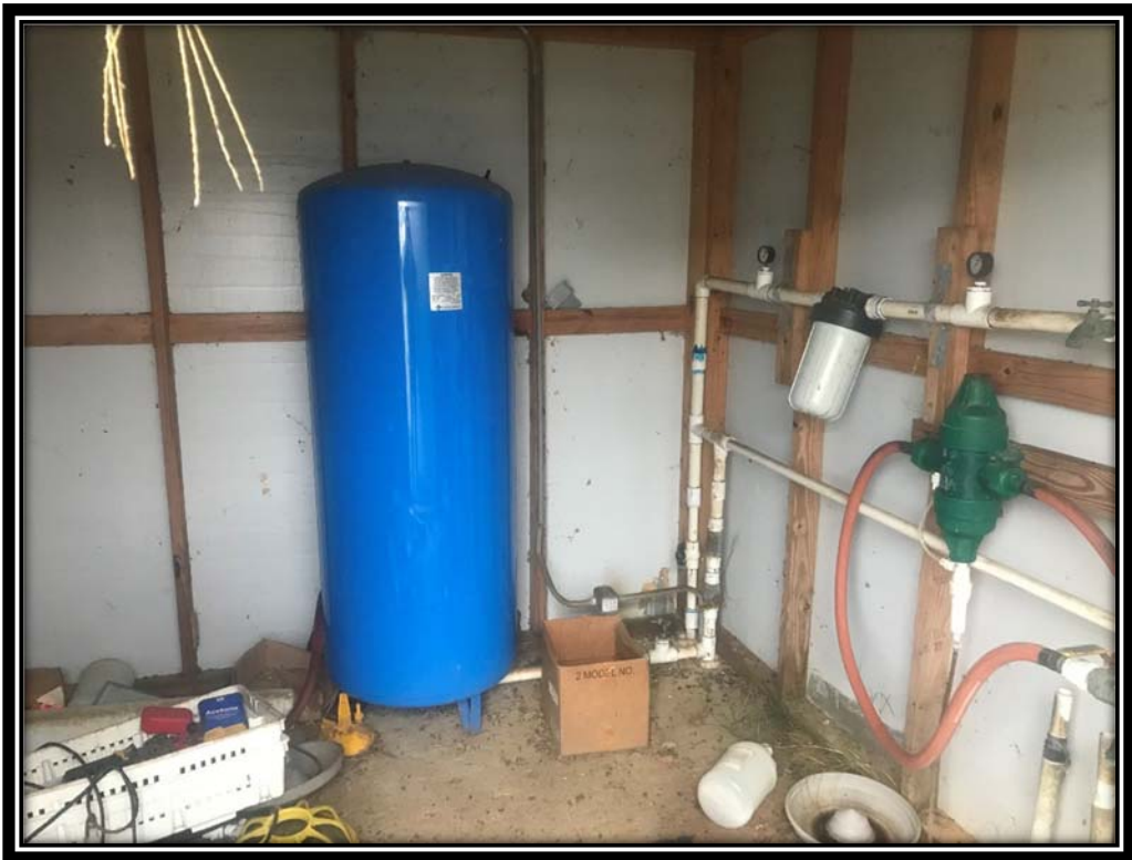
Blake Gamble-6729Z Water well Pump Shed
