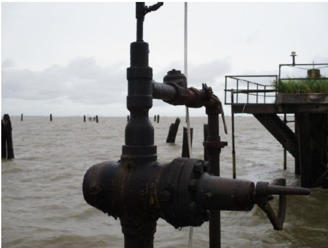
PICTURE OF CLOSED VALVES ON WELL HEAD
