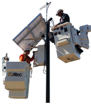
Pole-Mounted Battery Enclosure Solar Systems
