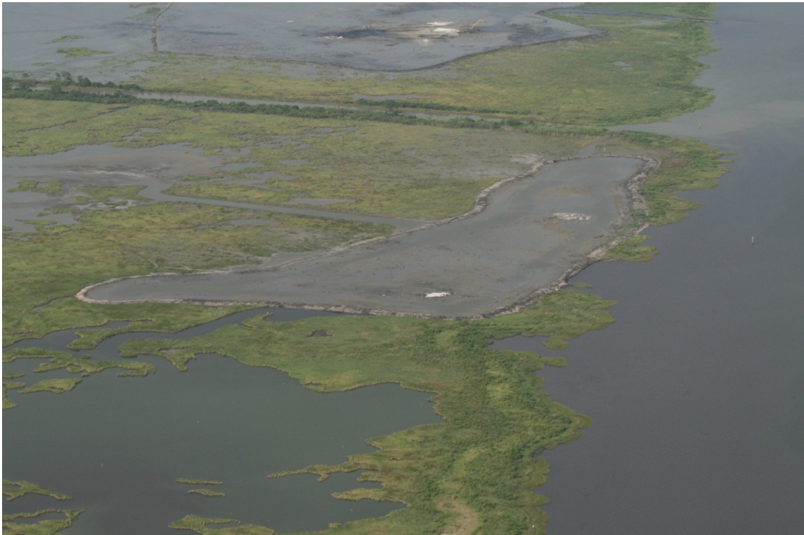
Showing perimeter diking
