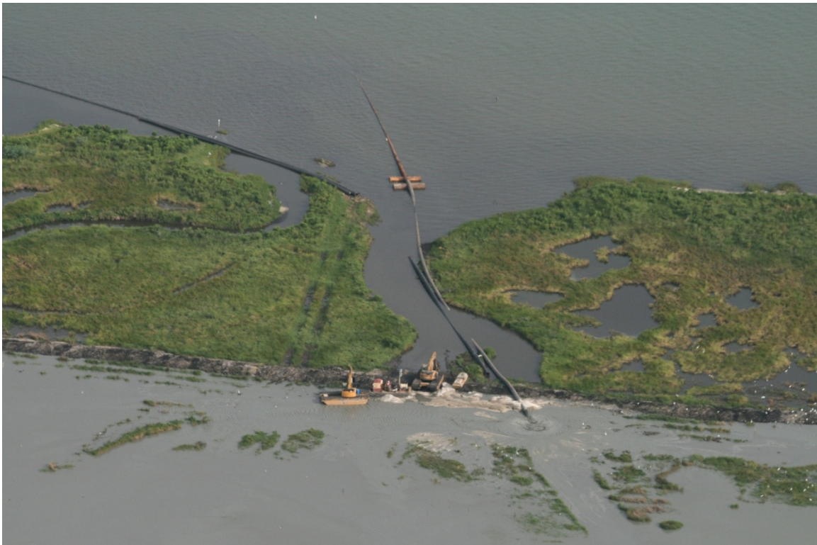
Placing dredged material
