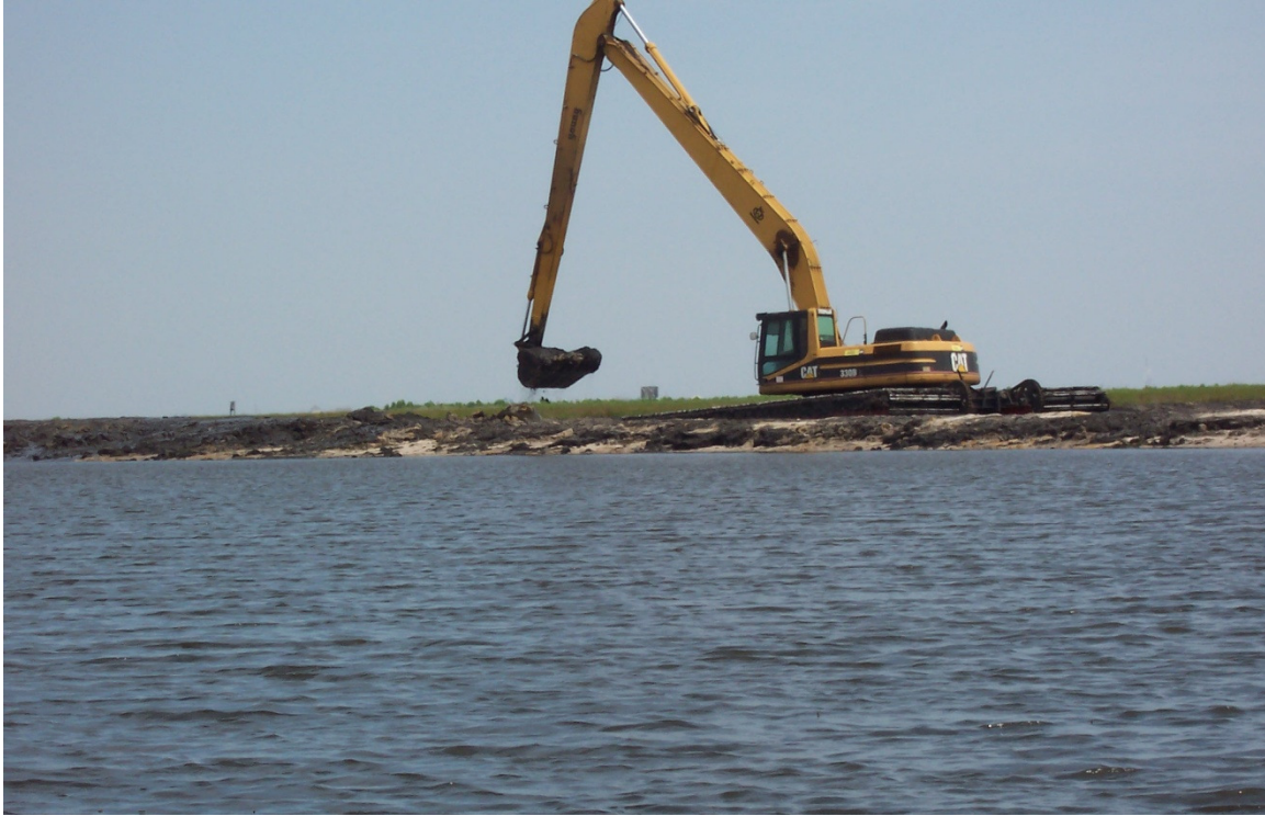
Construction Perimeter Diking GOOSE POINT/POINTE PLATTE MARSH FILL AREA C
