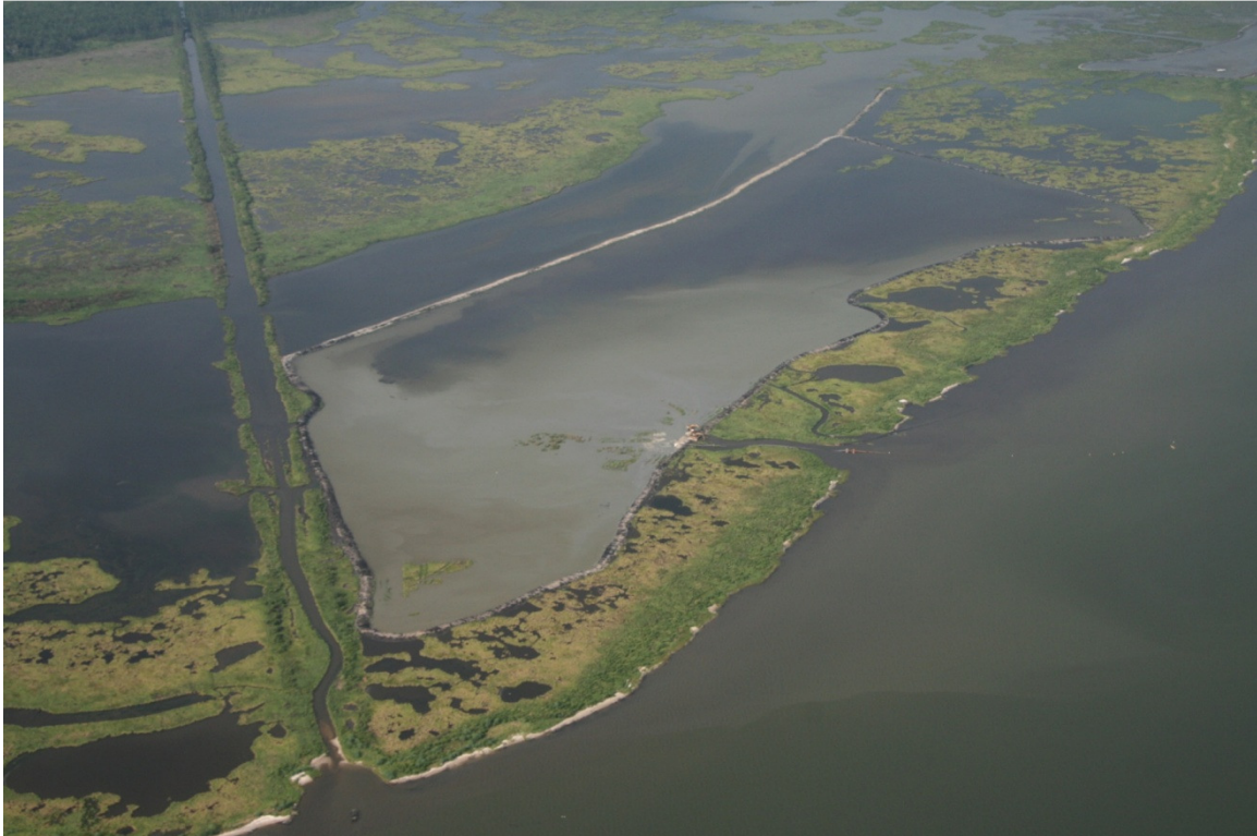
Showing perimeter diking FILL AREA D
