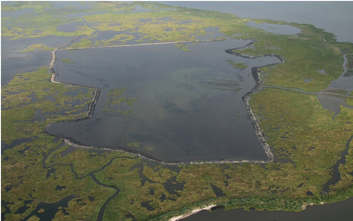
Showing perimeter diking
