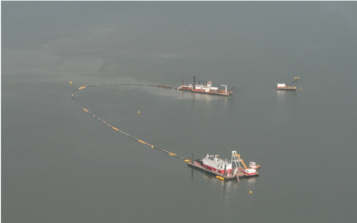
Dredge Borinquen (background), booster pump barge and anchor barge
