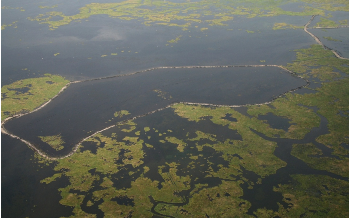
Showing perimeter diking FILL AREA B
