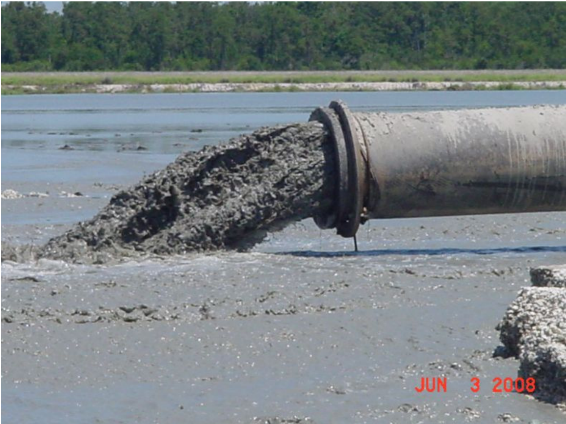
Placing dredged material
