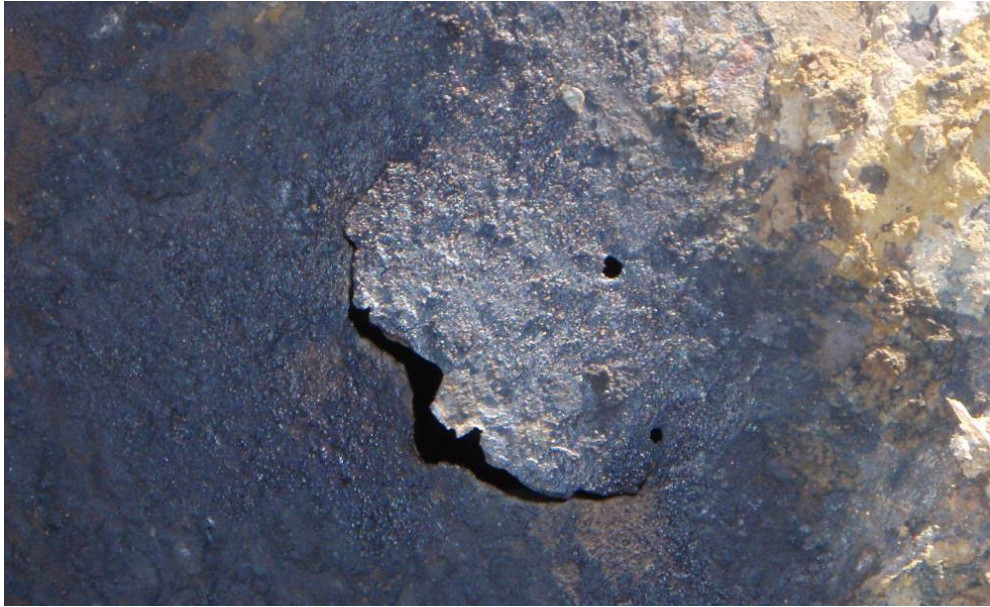
Figure 12. Failed Strainer (external view).
