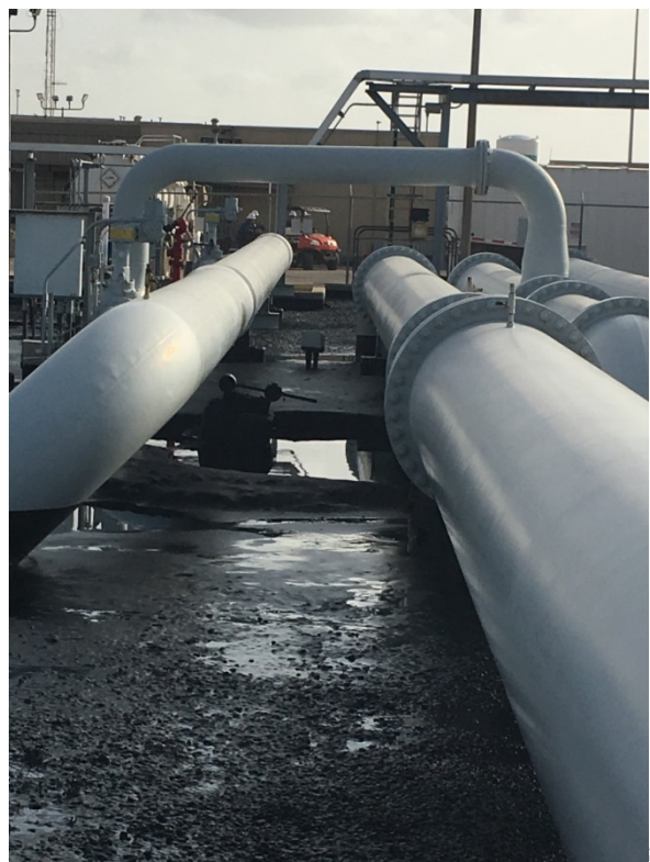
Figure 8. Crude Oil Pooling at Leak Location (Photo provided by Enterprise).
