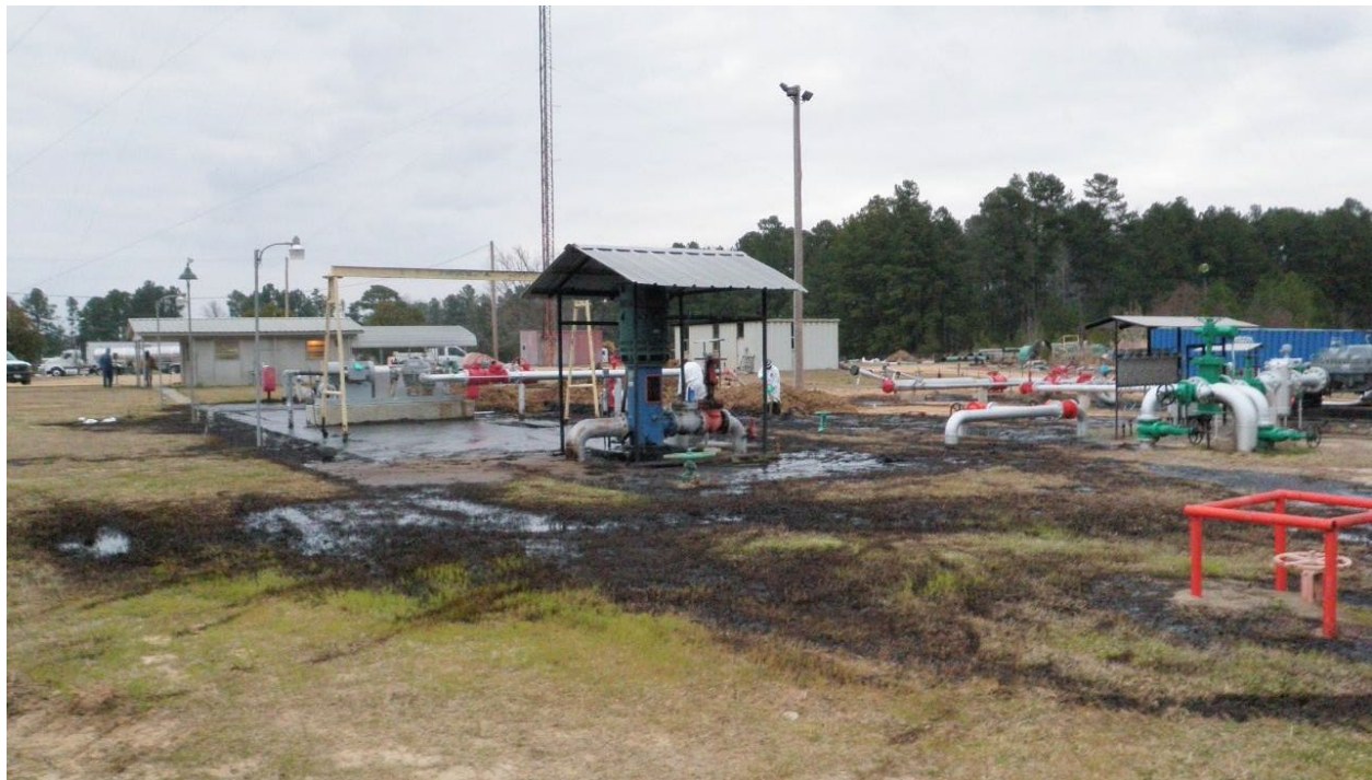
Figure 11. The release of oil was caused from a 12-inch underground pipe west of blue suction pump. Photo EPA.
