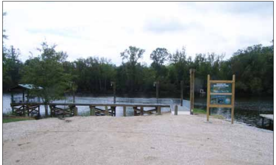
Phase II of the Big Alabama project included construction of this handicapped accessible fishing pier
