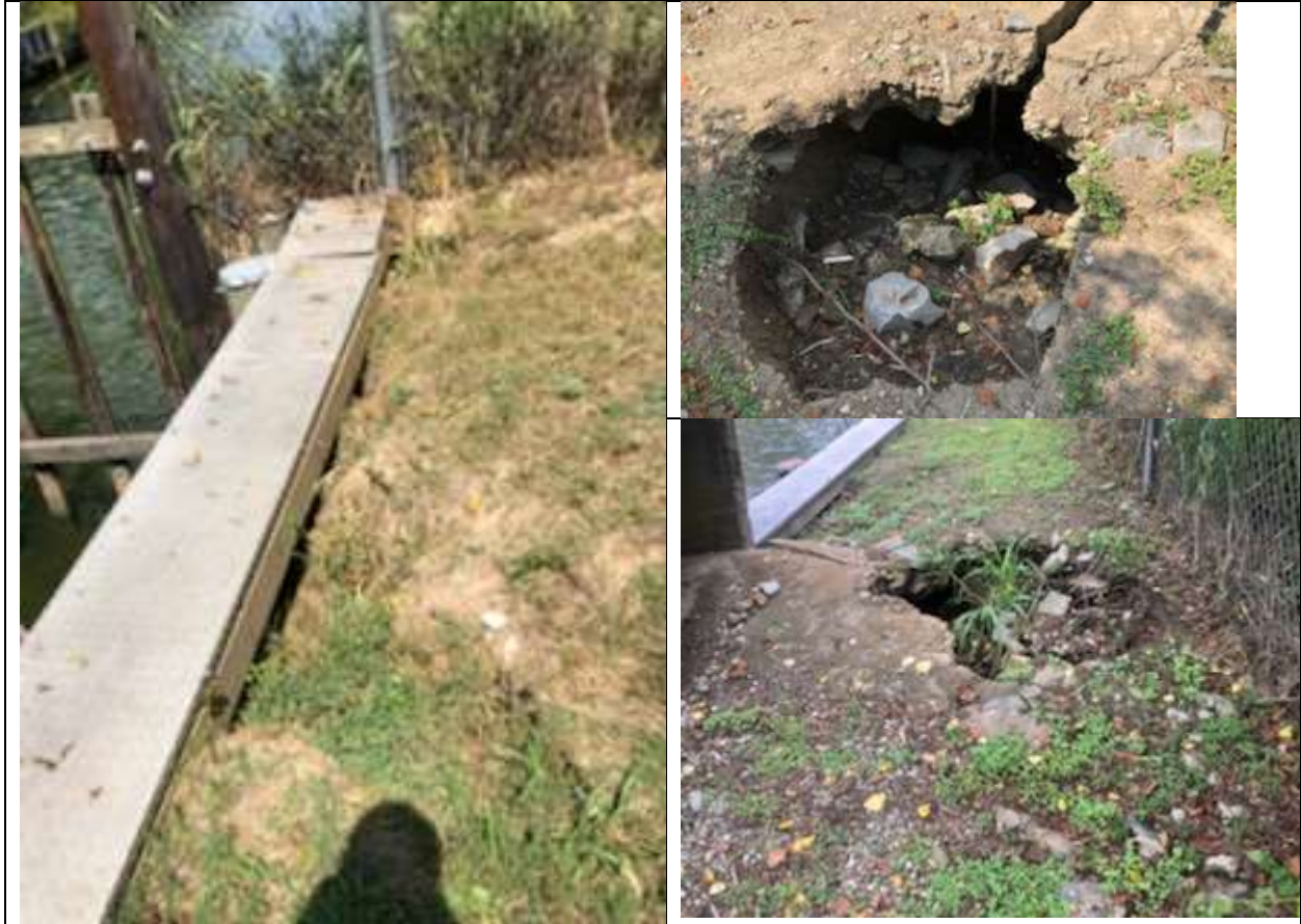
Figure 15: Photograph showing the erosion issues along the side of the control structure.
