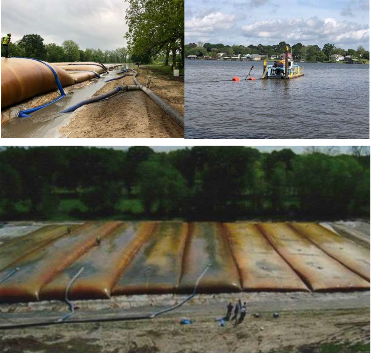
Figure 5: Photographs of the dredge operations, the suction dredge in False River (top left) geotextile dewatering tubes being filled (top right) and an aerial view of the dewatering site (bottom).
