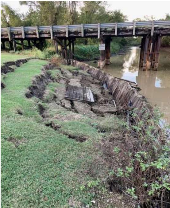
Figure 7: Photograph of the headwall Failure in Discharge Bayou
