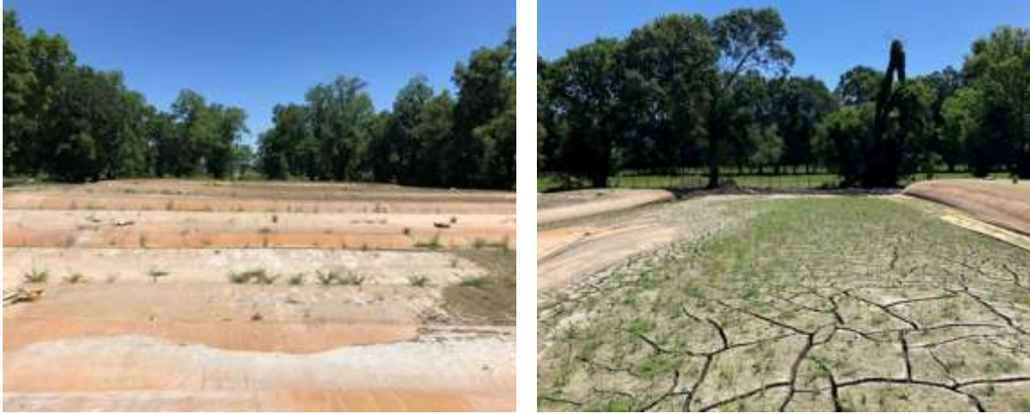
Figure 6: Photographs of the dewatering tubes (left) and dried sediment (right) at the dewatering site.
