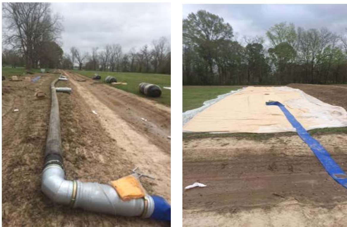
Figure 4: Photographs of the dredge pipe header (left) and geotextile dewatering tube (right) at the dewatering site.
