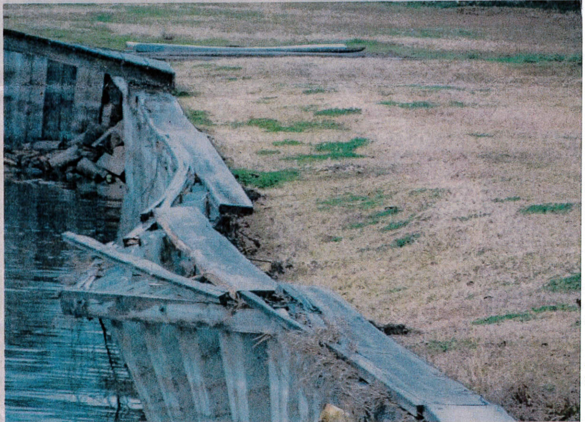
Despite what engineers told the attendees at a meeting on the drawdown hosted by the False River Civic Association many of them refused to believe the lower water level was not the cause of lakeside bulkhead failures.
