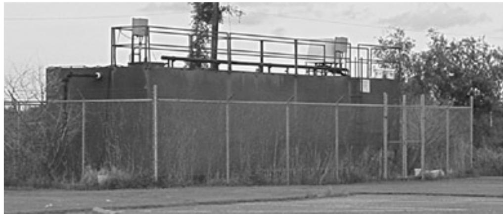
In addition to a pumpout system, Cypress Cove Marina has an above-ground sewage treatment plant on the premises. The tank has a capacity to treat approximately 24,000 gallons per day and is used to process sewage
