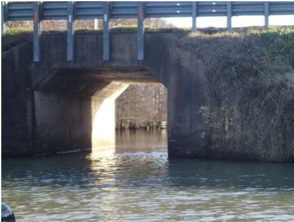
Photograph F6: View of the underside of the US Highway 65 bridge toward Tensas Bayou
