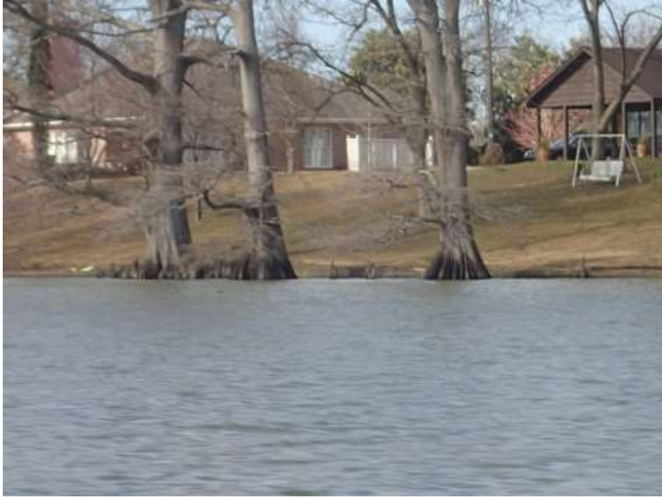
Photograph F15: Bulkhead located on inner east side of lake
