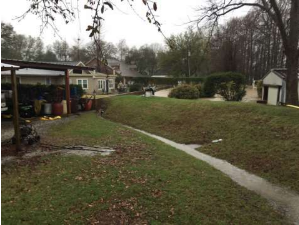
Photograph D1: Flooding at a residence on Island Point drive, Lake Providence
