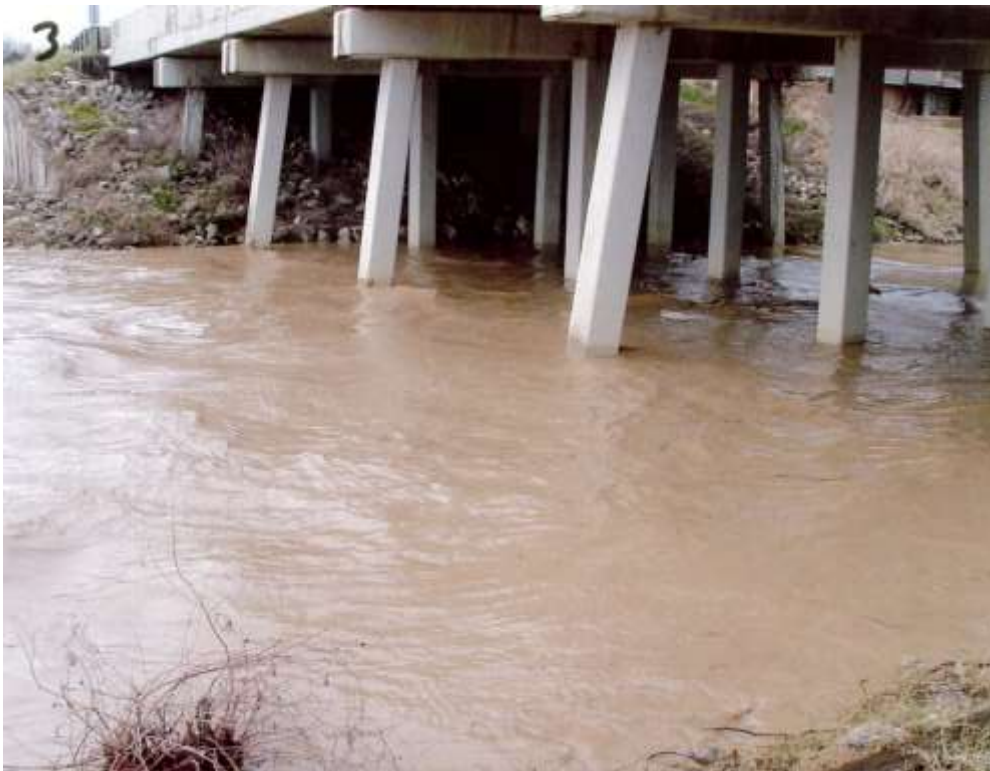
Photograph E3: Baxter Bayou outfall. Note water turbidity.
