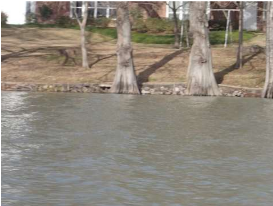
Photograph F16: Bulkhead and riprap located on inner east side of lake
