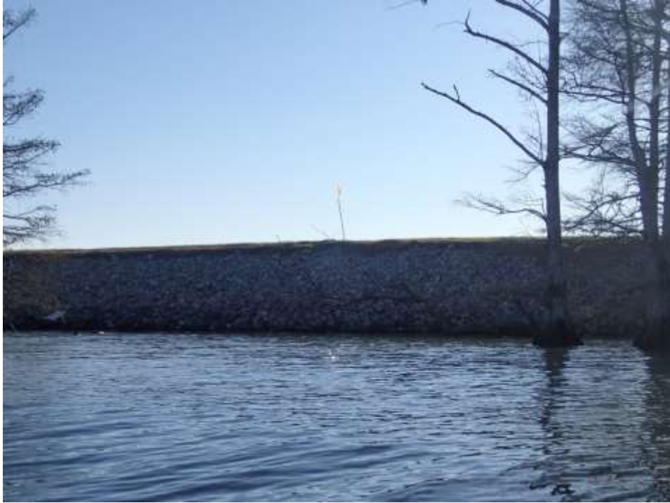
Photograph F21: Riprap revetment located along U.S. Highway 65 on western side of the lake
