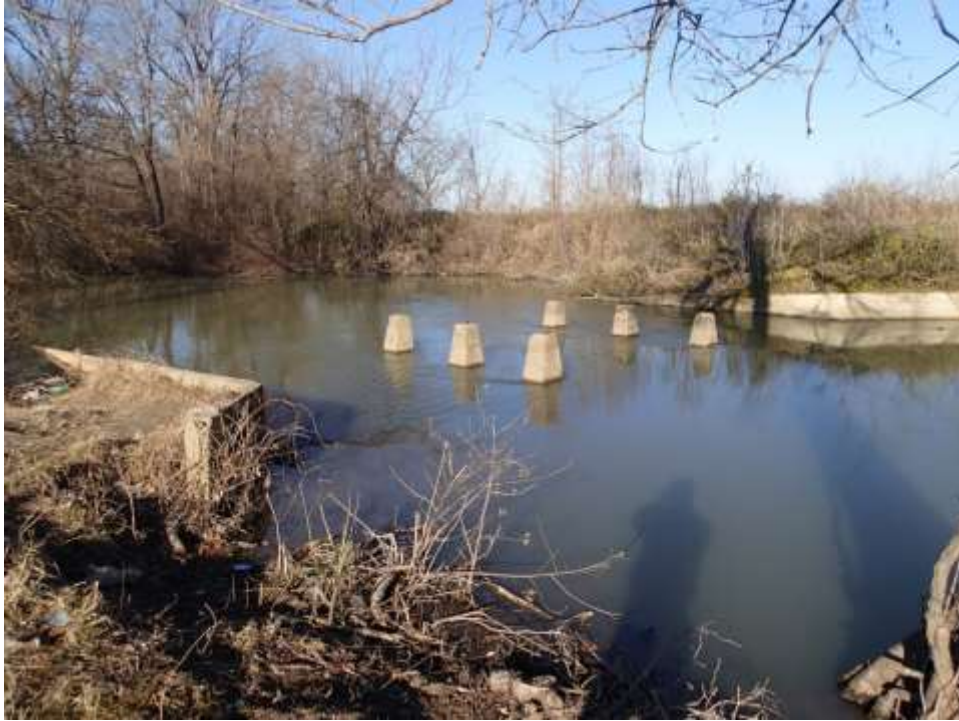
Photograph F13: Weir located on Tensas Bayou
