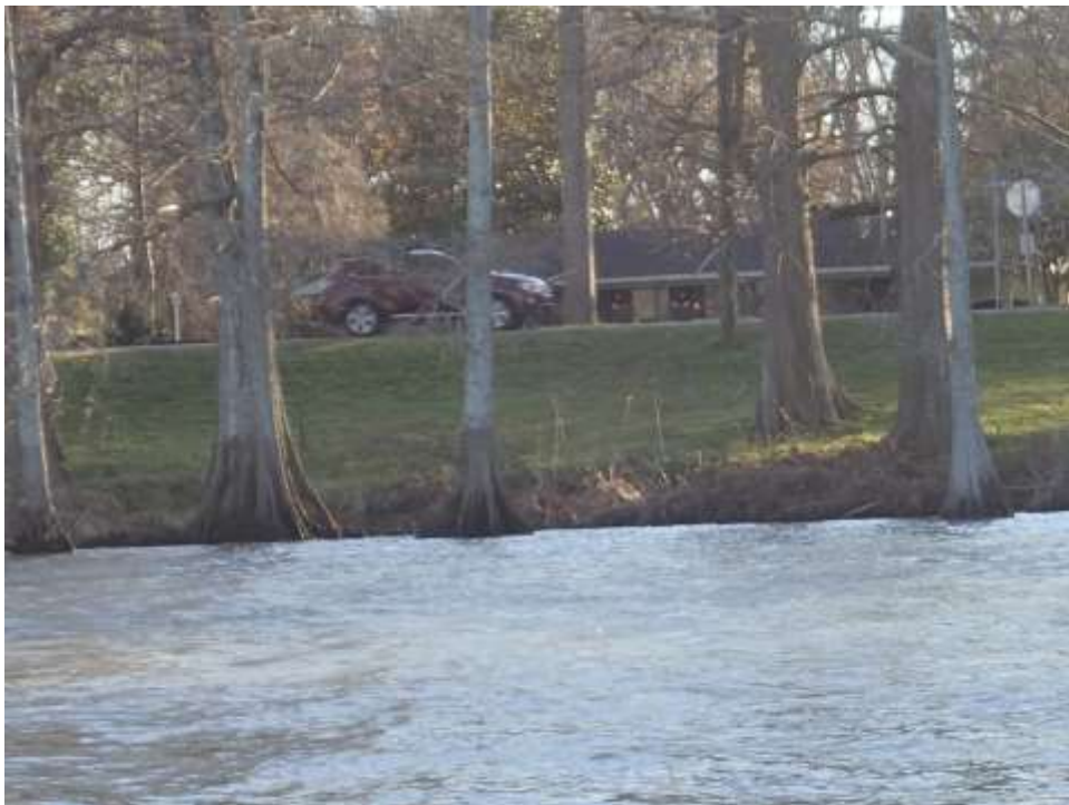
Photograph F26: Cypress tree shoreline along U.S. Highway 65 close to Grant's Canal showing high water marks on the trees.
