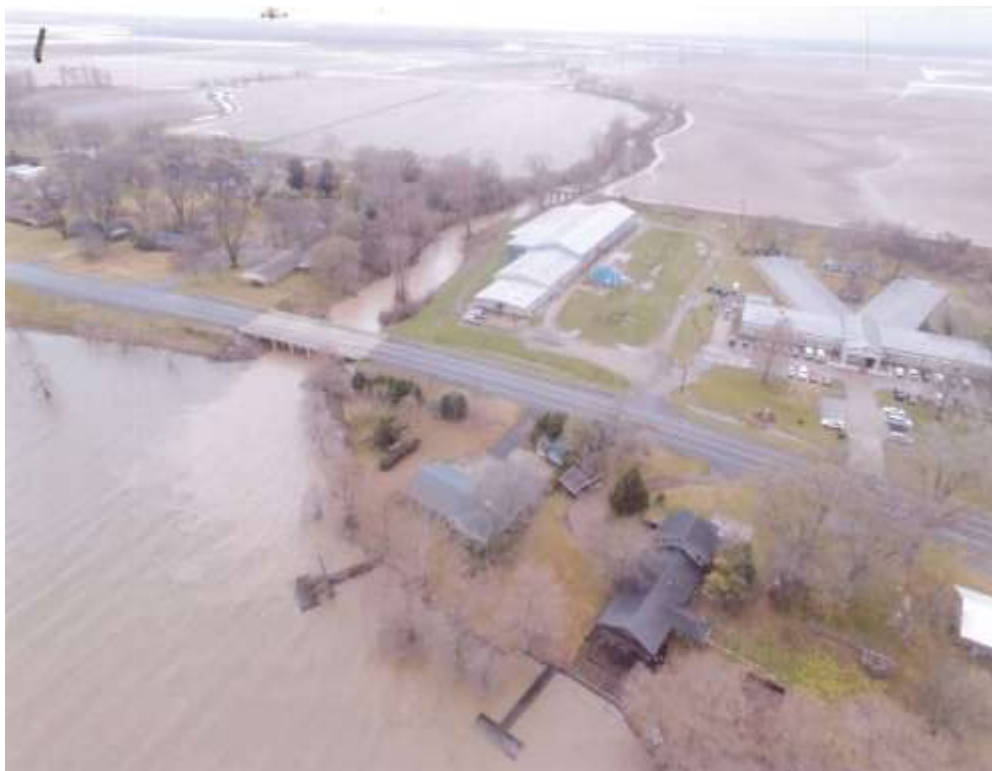
Photograph E1: Baxter Bayou outfall
