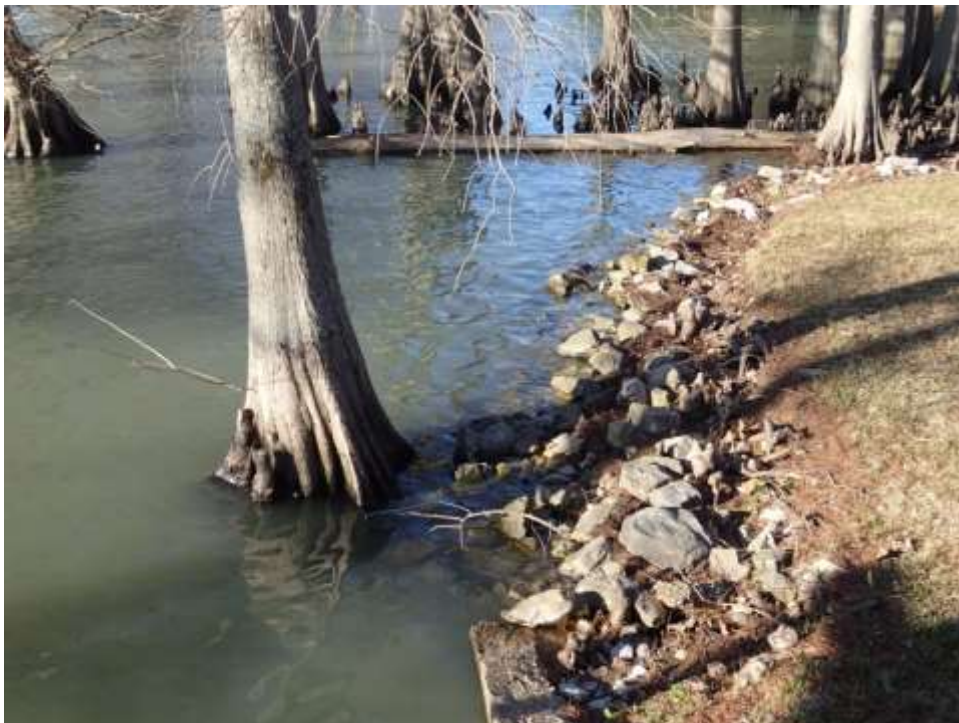
Photograph F20: Riprap revetment located on inner east side of lake
