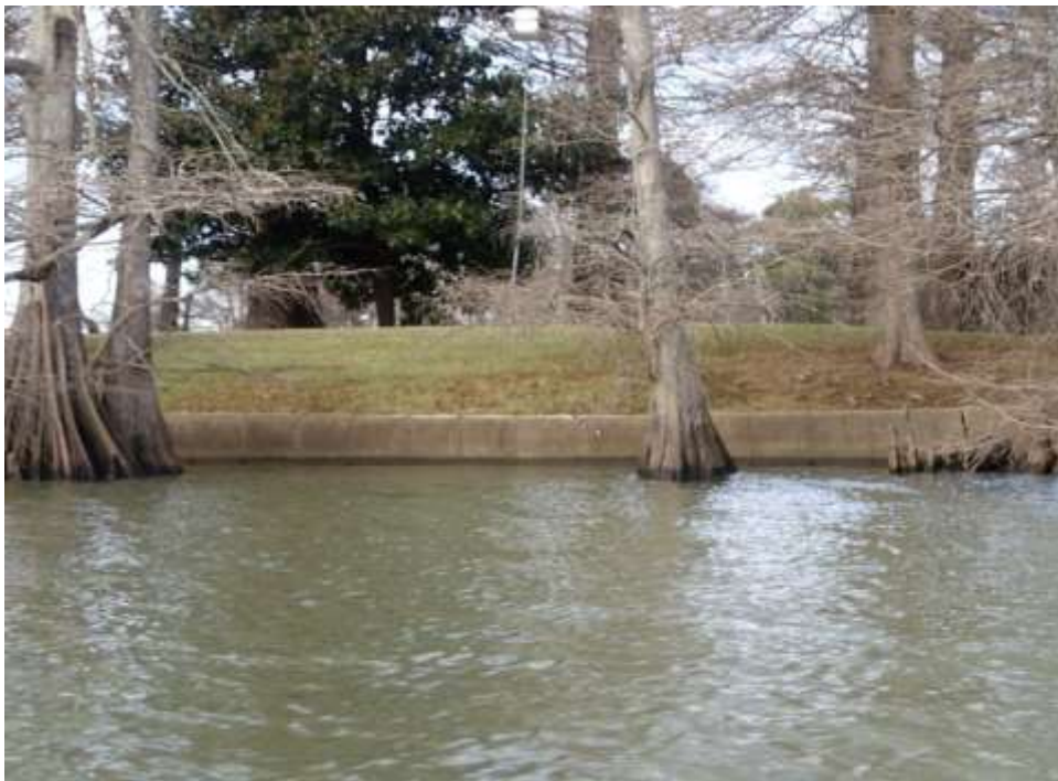
Photograph F14: Bulkhead across from airport landing on Chute
