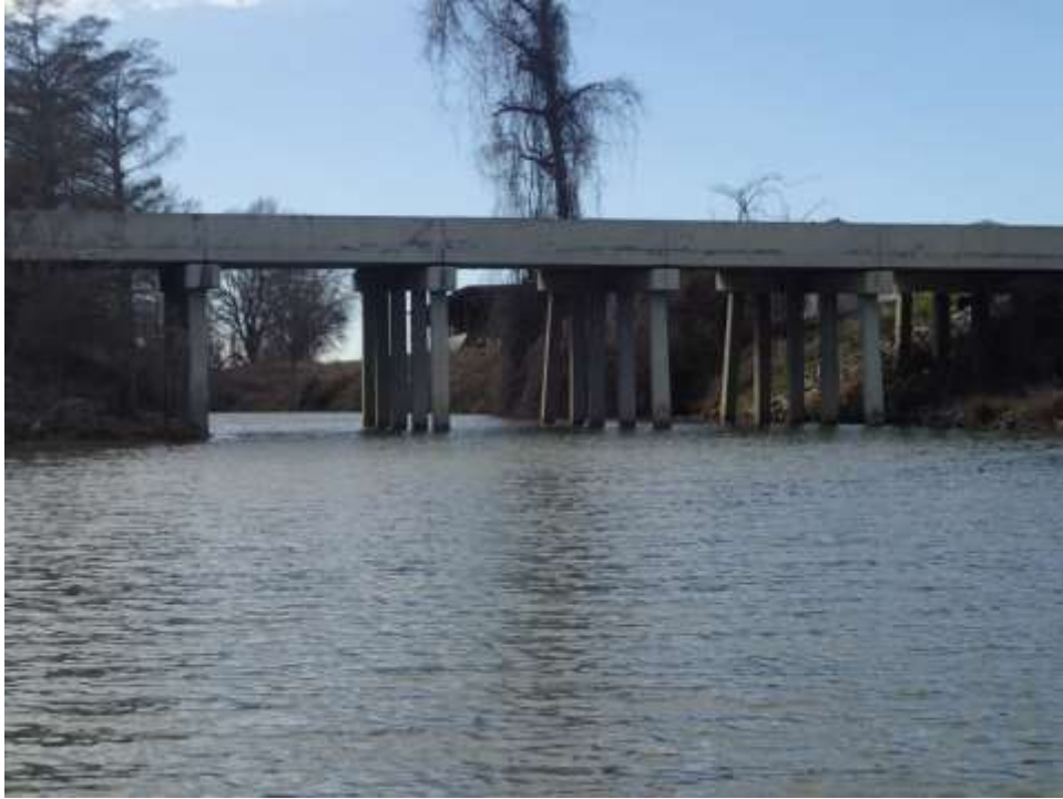
Photograph F27: Baxter Bayou Bridge along U.S. Highway 65
