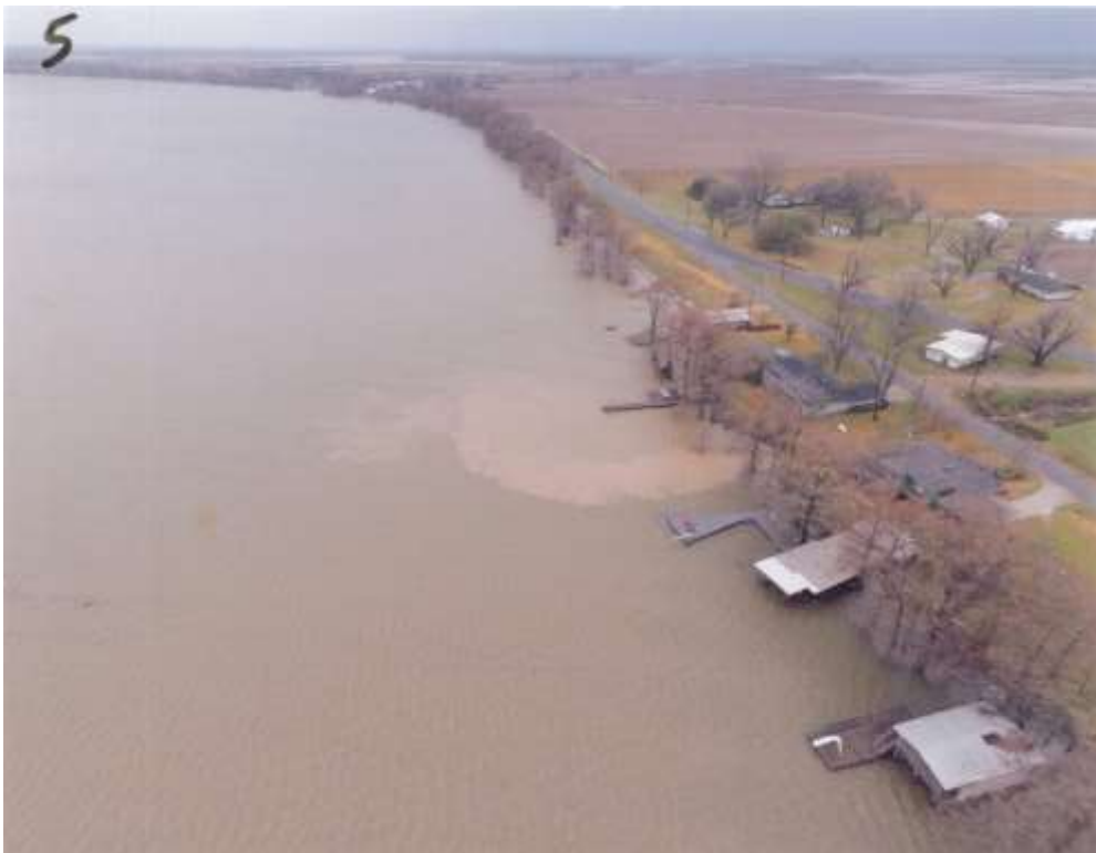
Photograph E5: Drainage ditch outfall south of Black Bayou
