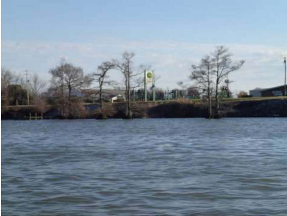
Photograph F23: Riprap revetment along U.S. Highway 65
