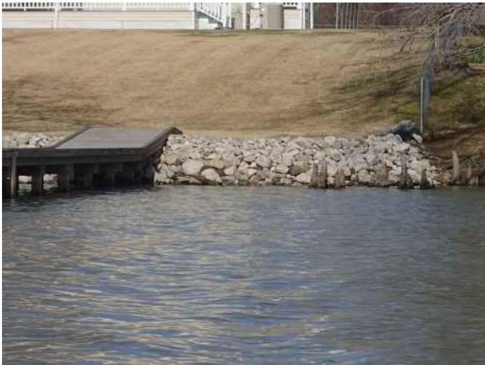
Photograph F18: Riprap revetment located on inner east side of lake
