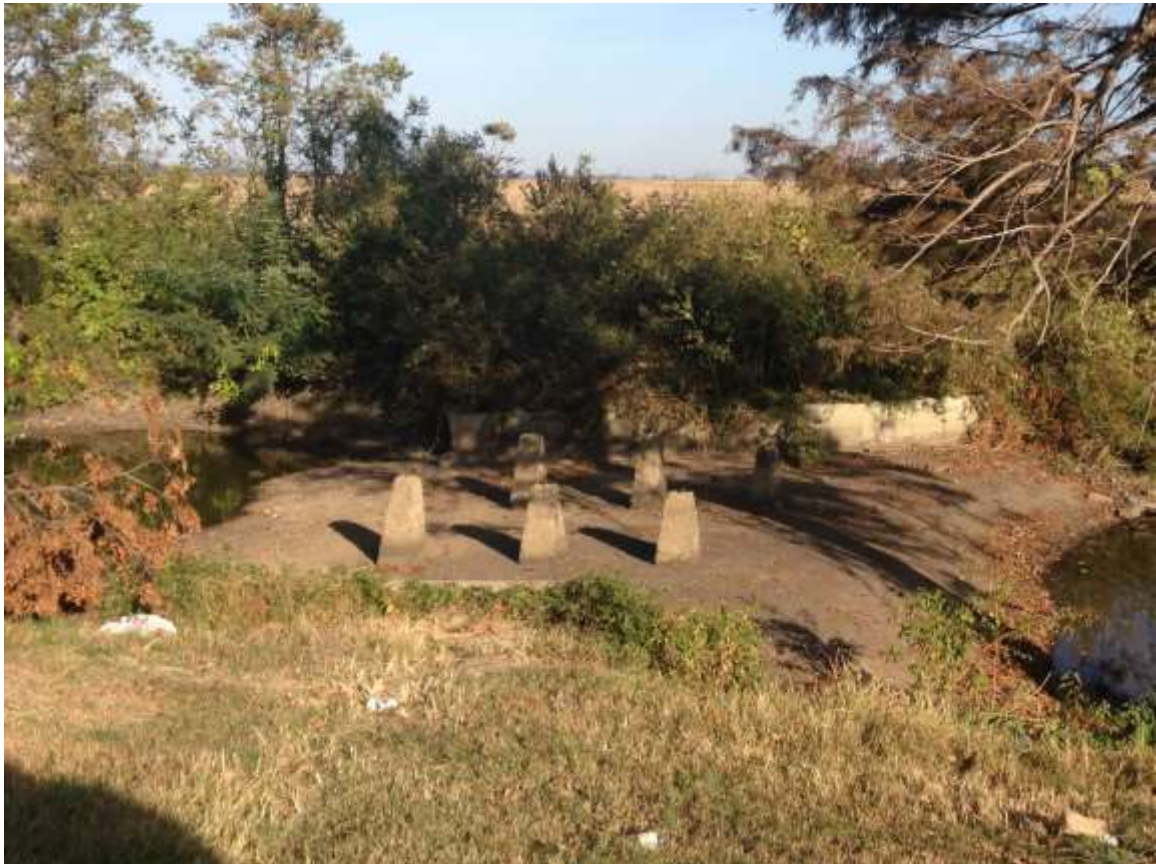
Figure 7: Tensas Bayou weir. The Google Earth™ photograph (top) was taken on 11/15/12; the profile view (bottom) of the structure on 10/21/15
