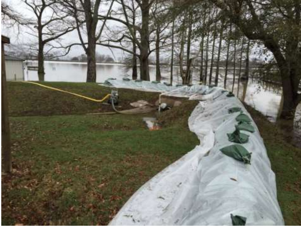
Photograph D9: Flooding at a residence on Island Point drive, Lake Providence
