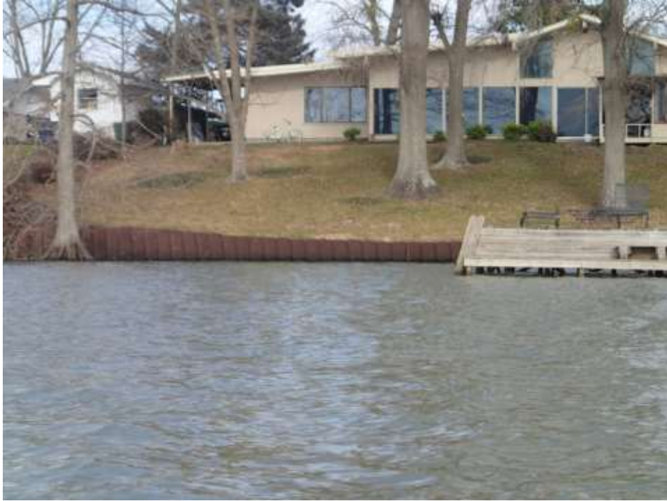
Photograph F19: Bulkhead located on inner east side of lake
