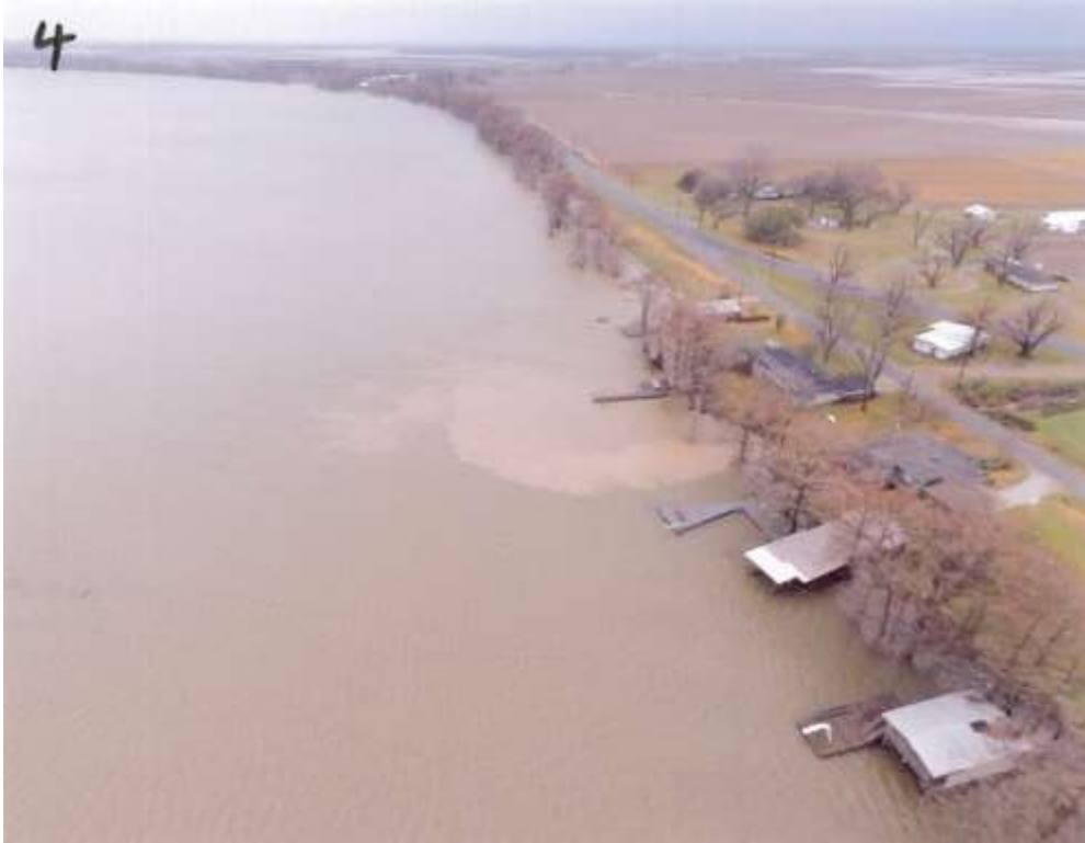
Photograph E4: Drainage ditch outfall south of Black Bayou
