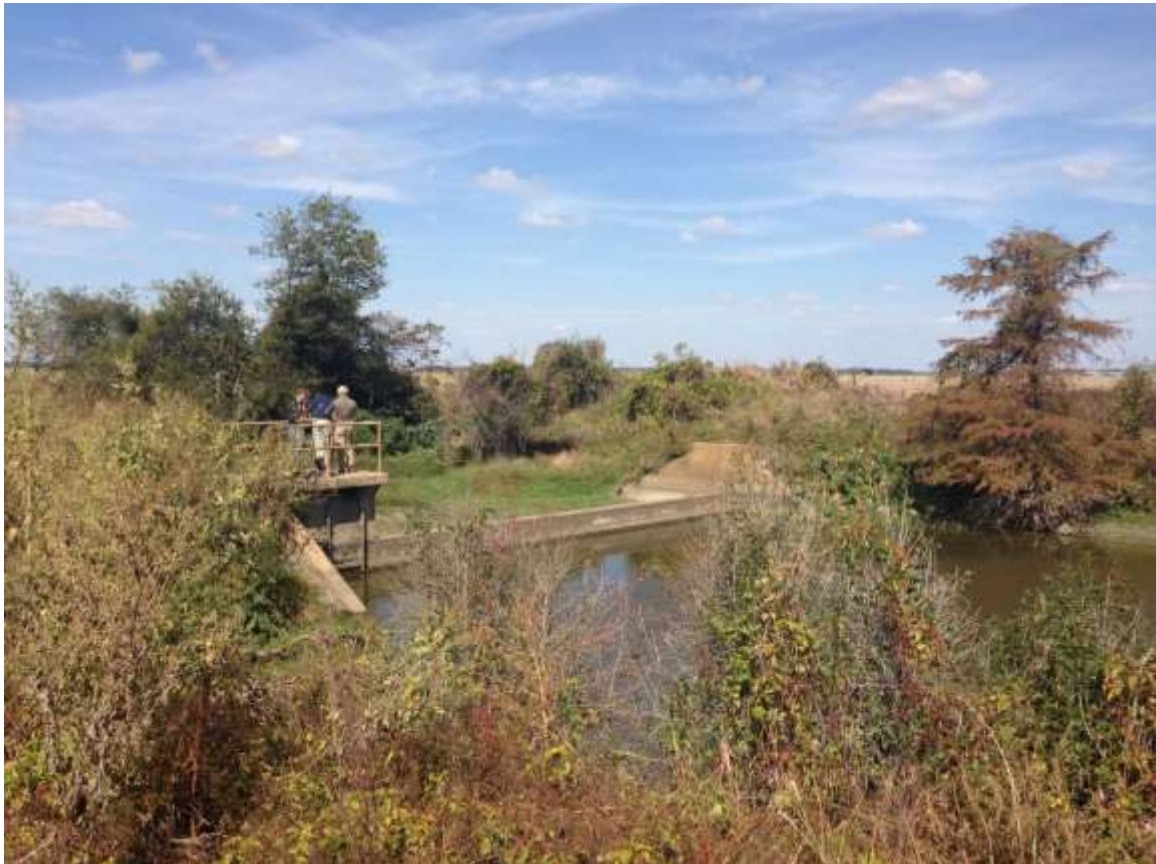
Figure 8: Baxter Bayou control structure.
