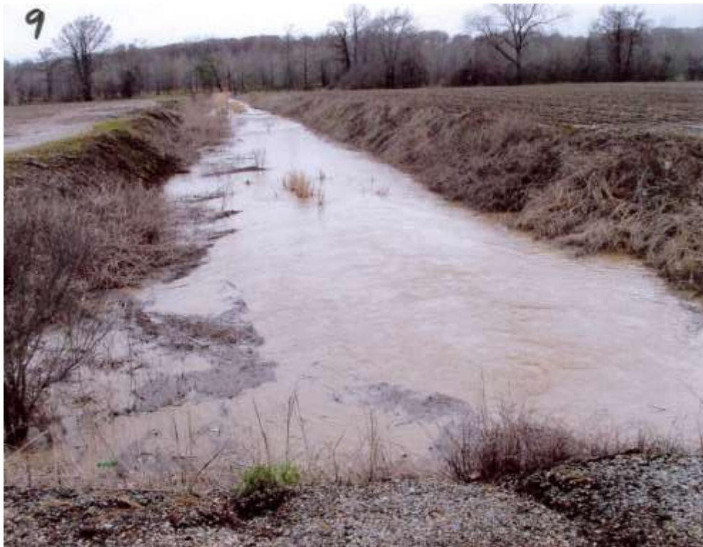
Photograph E9: Drainage ditch flowing into Bayou Providence
