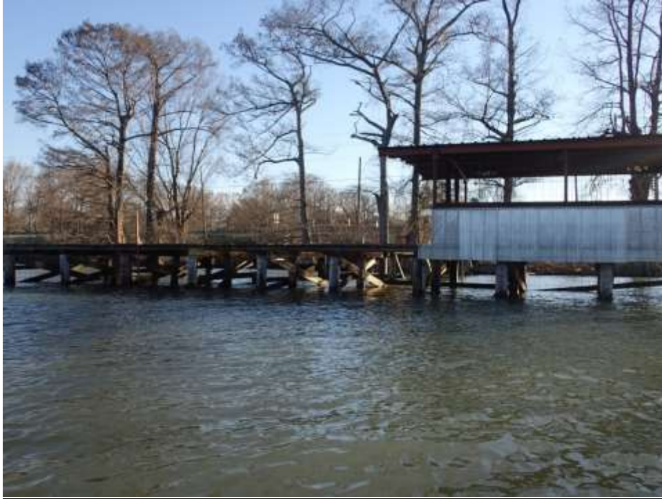
Photograph F5: Old swimming pier where the new LGS data gage has been installed
