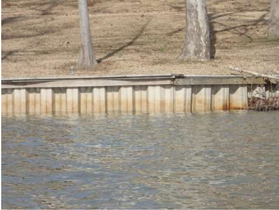
Photograph F17: Bulkhead located on inner east side of lake
