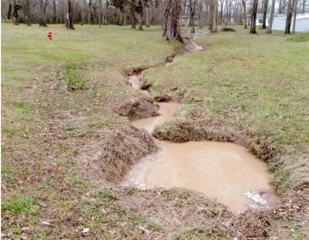
Photograph E18: Rill erosion near the North Flat
