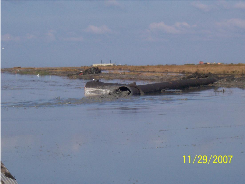
Dedicated Dredge Project at Point Au Fer (6 Months Post-Construction)
