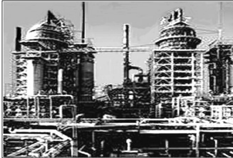
Exxon-Mobil Refinery - Baton Rouge
