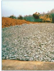
**Construction entrances should be flared to allow for turning vehicles.**
