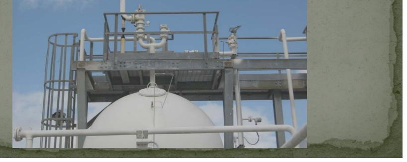
Aboveground breakout tanks that are constructed or significantly altered according to API Standard 2510 after October 2, 2000 must have an overfill protection system installed according to section 5.1.2 of API Standard 2510.
