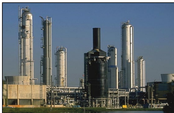
Promix Fractionation Plant
