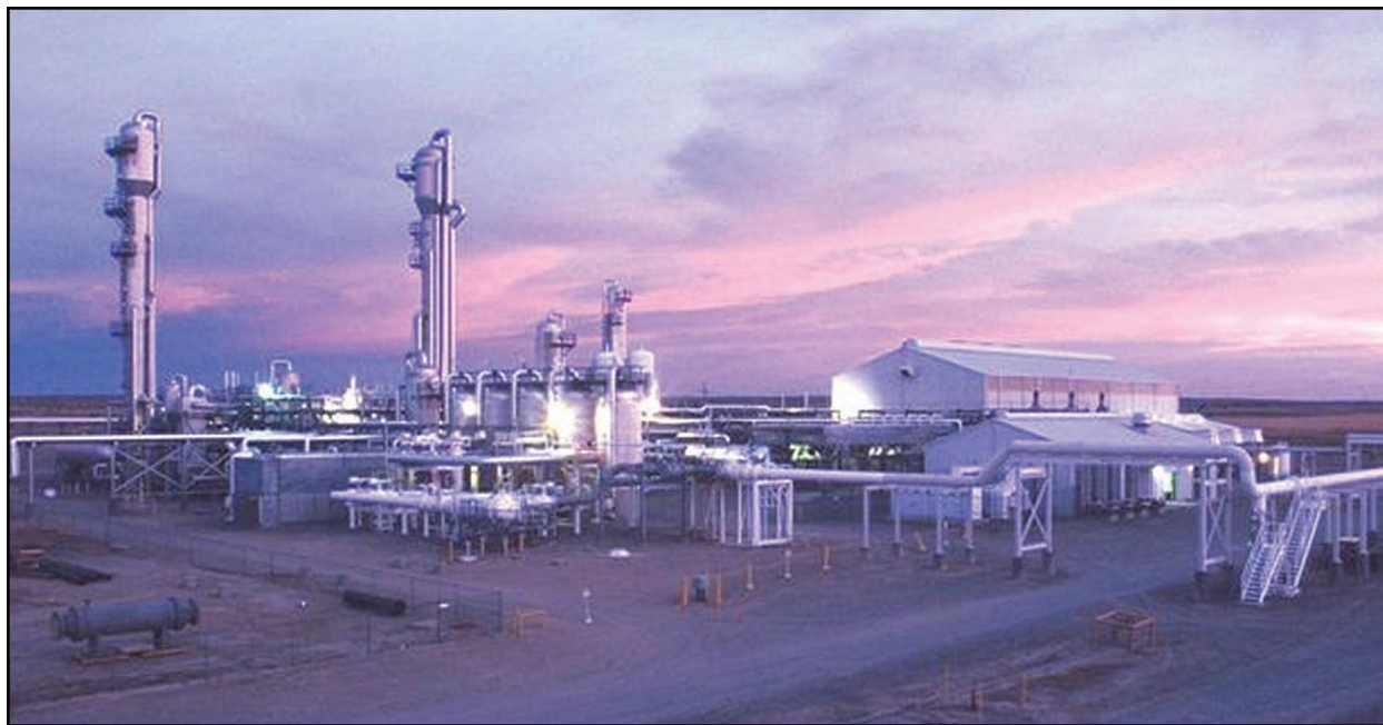
Enterprise Natural Gas Processing Plant
