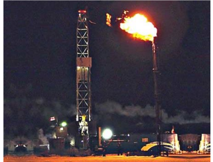
Gas flare from well testing
