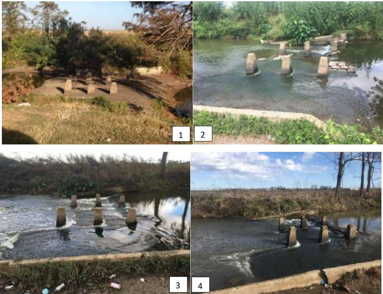
Figure 1: Condition of the Tensas Bayou weir in Oct 2015 (1), August 2020 (2), October 2020 (3) and March 2021 (4). Notice the cement bags installed in August 2018 to prevent erosion and pass of the structure.
