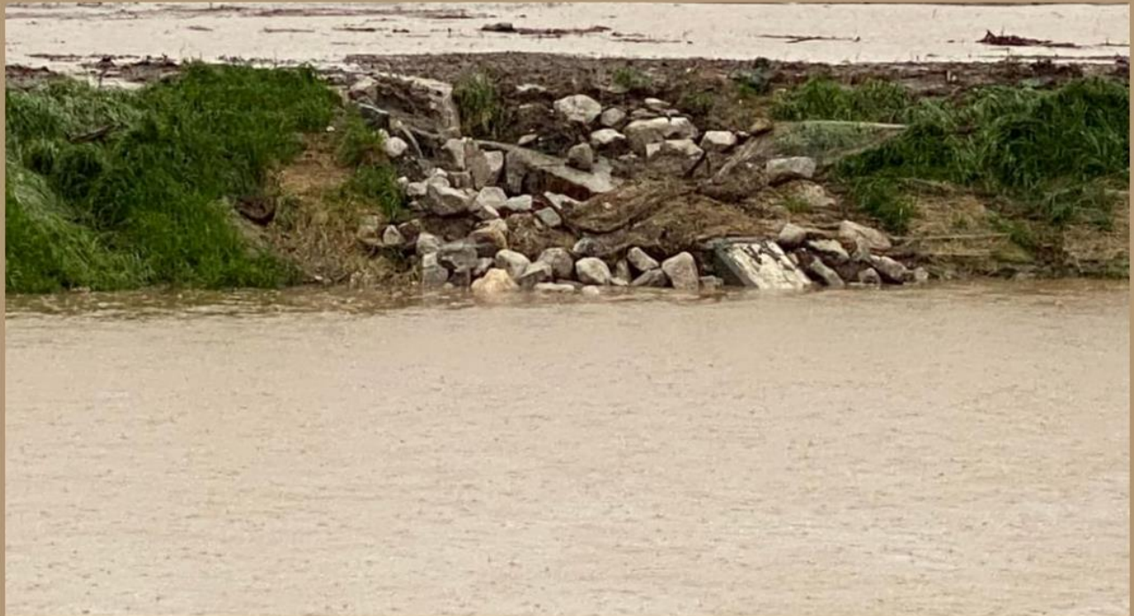
Photo A1: Picture of the Tensas weir prior and during the April 2024 flood. Note damage to the weir embankment armoring. Photo taken by Larry Brock
