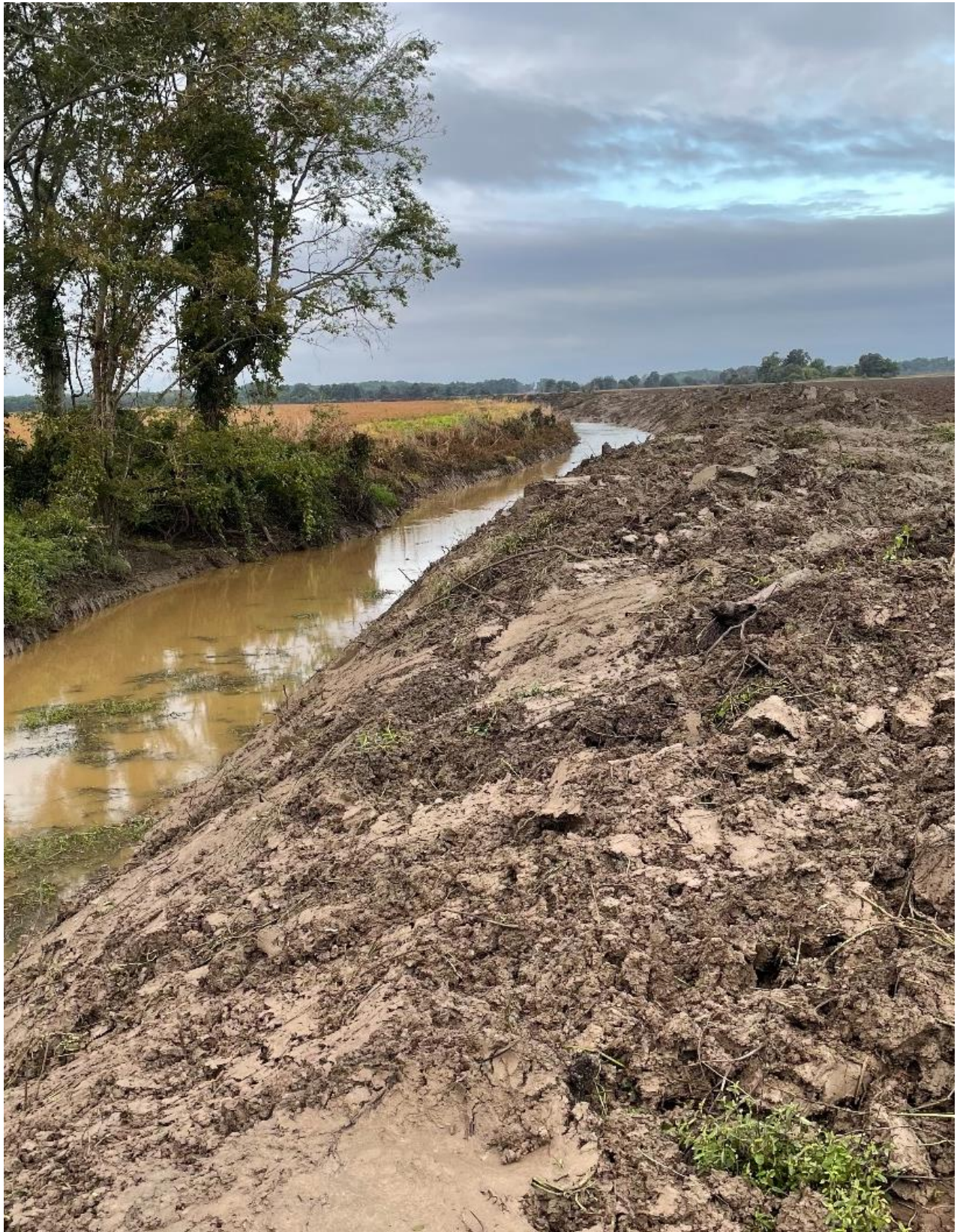
Photo B3: After picture taken on September 10 th following a 3-in rain. This photo is showing areas cleared on Baxter Bayou facing towards the structure. Photo taken on 9/10/21 by Bo Holt.
