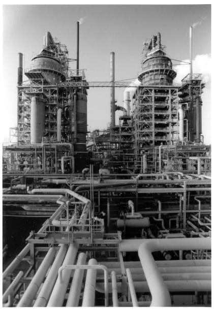
Catalytic cracking technology invented at Exxon Baton Rouge in 1942 helped win WWII. It remains industry standard. Photo courtesy Exxon Public Affair
