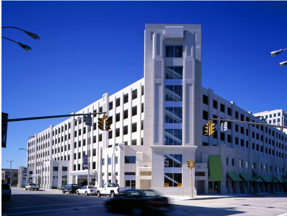
Galvez Parking Garage
