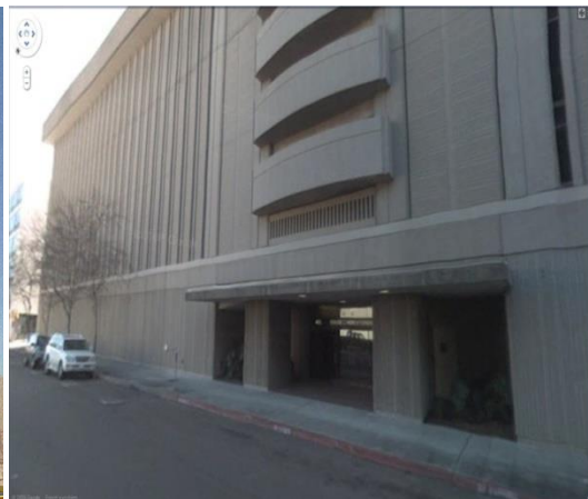
Entrance to Chase Tower North at 450 Laurel Street
