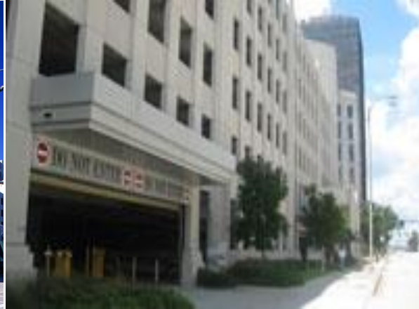
Garage Entrance on North Street
