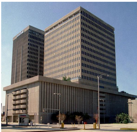
Location of CPRA: Chase Tower North
