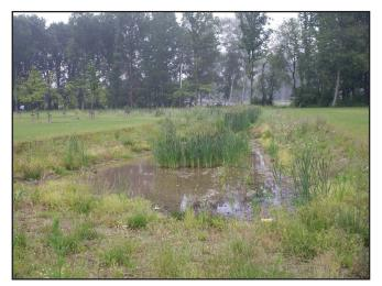
1. Store and detain floodwater. Incorporate pre-existing low-lying areas, natural drainage swales or streams into the layout of a subdivision or whole neighborhood. These areas are used to store or detain flood water in the event of heavy rain or storm. The area may be seasonally dry in the case of lowlying ground depression, or the area
