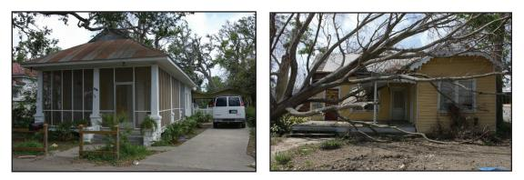
**Figures 6-18 and 6-19.** Healthy, well-maintained trees can help mitigate the effects of hurricanes and help protect nearby structures by reducing wind flow. However, poorly maintained or diseased trees located too close to a home can cause serious damage (Photos by B. Kennedy, 2006).
