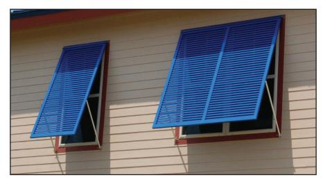
**Figure 6-13.** Permanently installed Bahama shutters provide light and shade when opened and protection from wind-borne debris when closed (Photo by D. Hwang, 2007).
