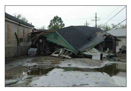
**Figure 6-2.** Air pressure and uplift worked to detach this roof from the rest of the structure. These types of forces can be mitigated against through the use of stronger connections, such as hurricane clips (Photo by B. Kennedy, 2006).
