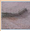
Hay bales offer temporary sediment filtration and can slow runoff velocity.
