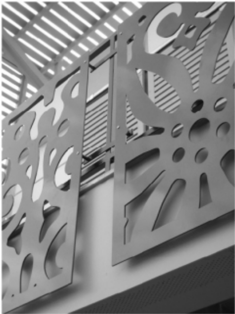
Detail of aluminum panel on front porch
