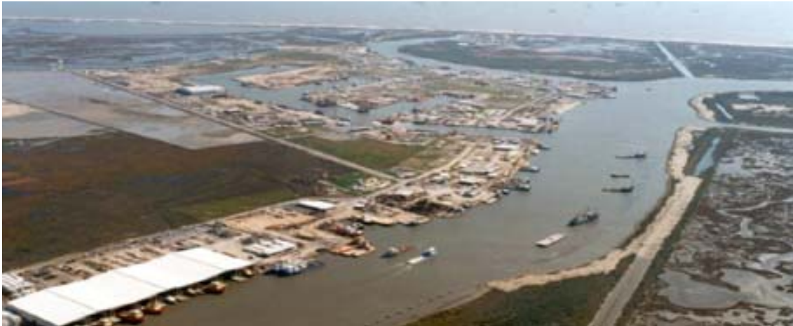
Aerial view of Port Fourchon, America's Energy Port
