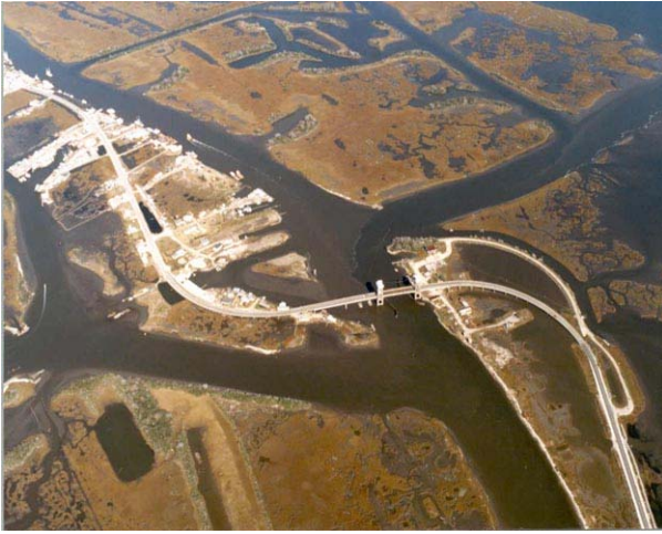
Leeville Bridge the “weakest link” in the supply chain to Port Fourchon.
