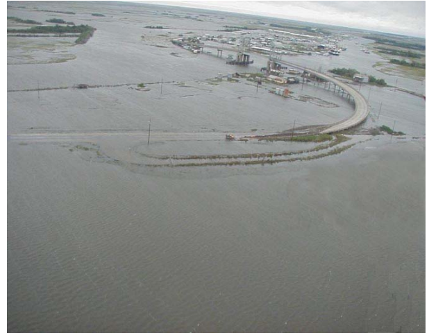
LA 1 and Leeville after a minimal Tropical Storm.
