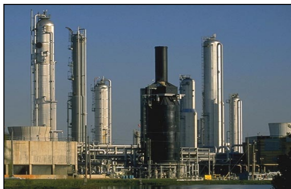
Promix Fractionation Plant
