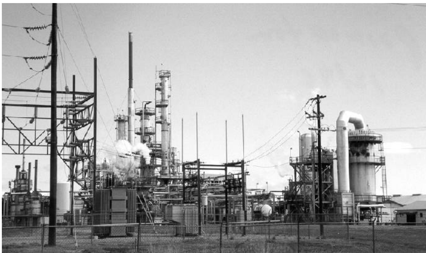
Calumet Refinery at Princeton. 1996 photo by Al Troy, La. Dept of Natural Resources
