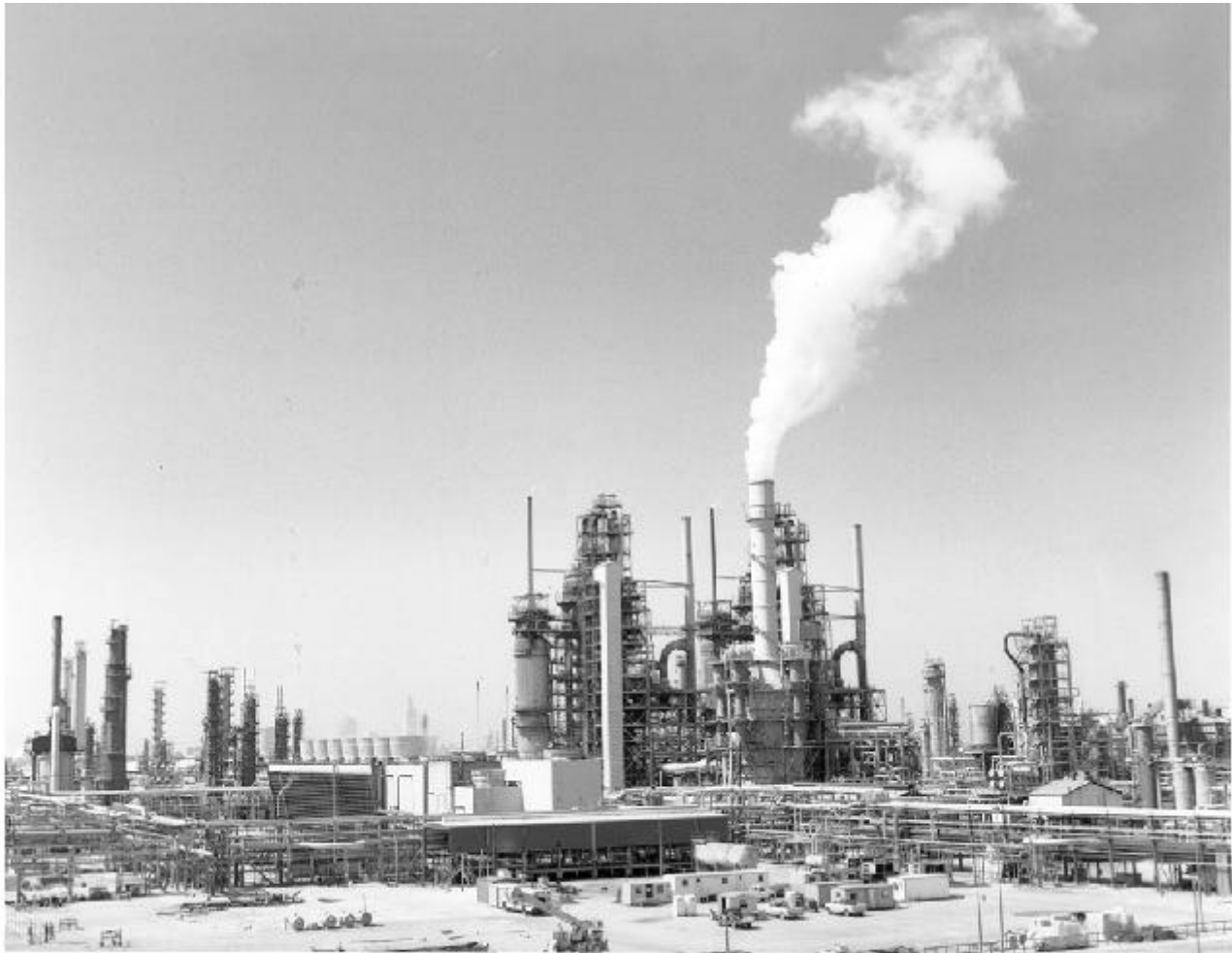
Exxon Baton Rouge looking Southwest. Plume is coming from wet gas scrubber. Photo courtesy Exxon Public Affairs.
